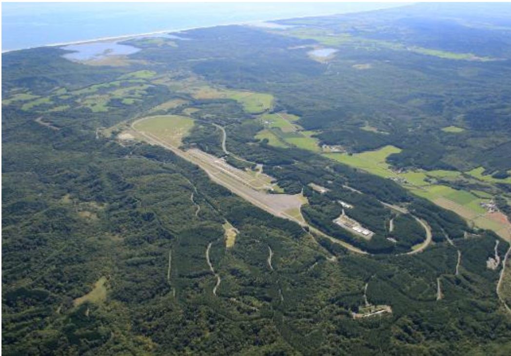
Hokkaido Toyokoro Proving Ground
